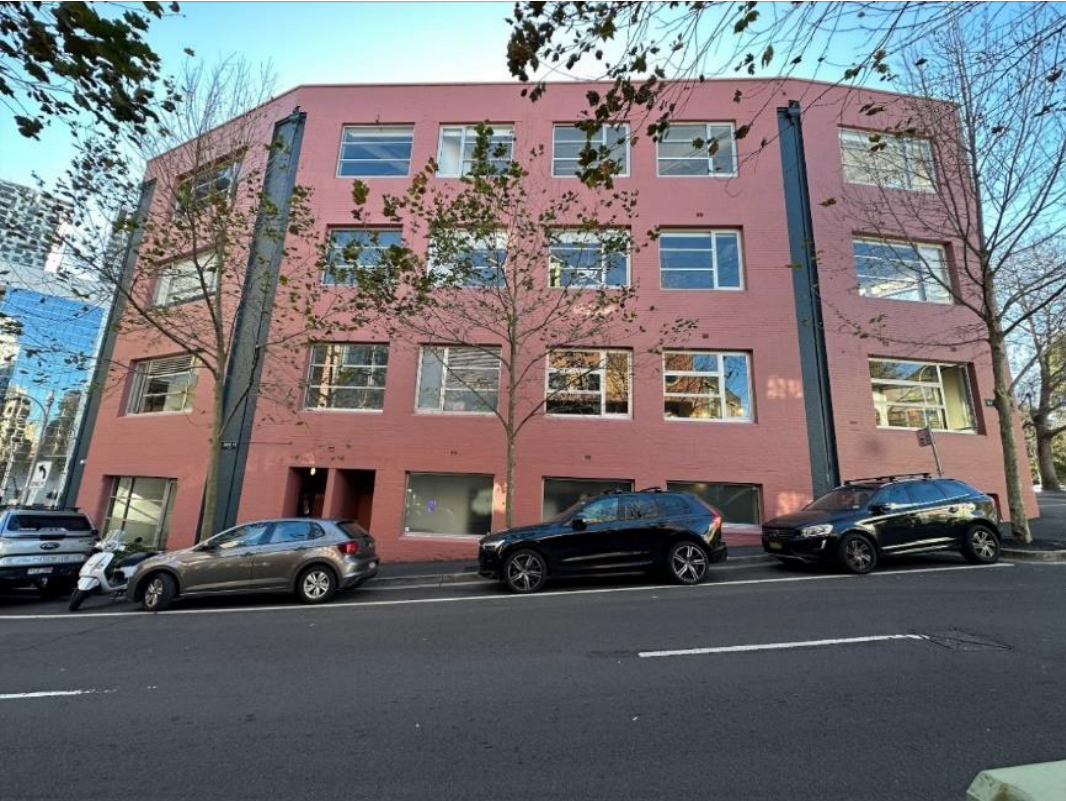
Figure 3. The existing building at 85-93 Commonwealth Street, looking north-east from Hunt Street
