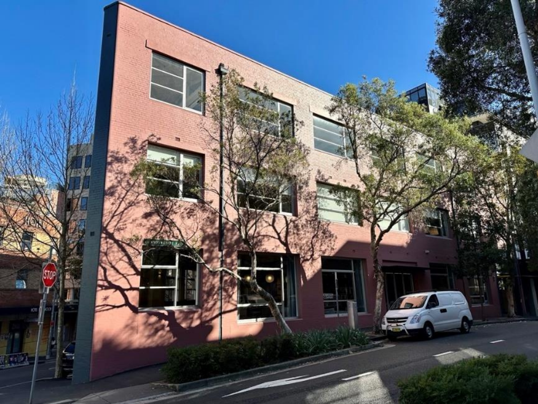
Figure 2. The existing building at 85-93 Commonwealth Street, looking west from Commonwealth Street
